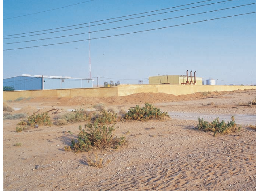
Thadeq power plant Providing Raghbah with electricity
