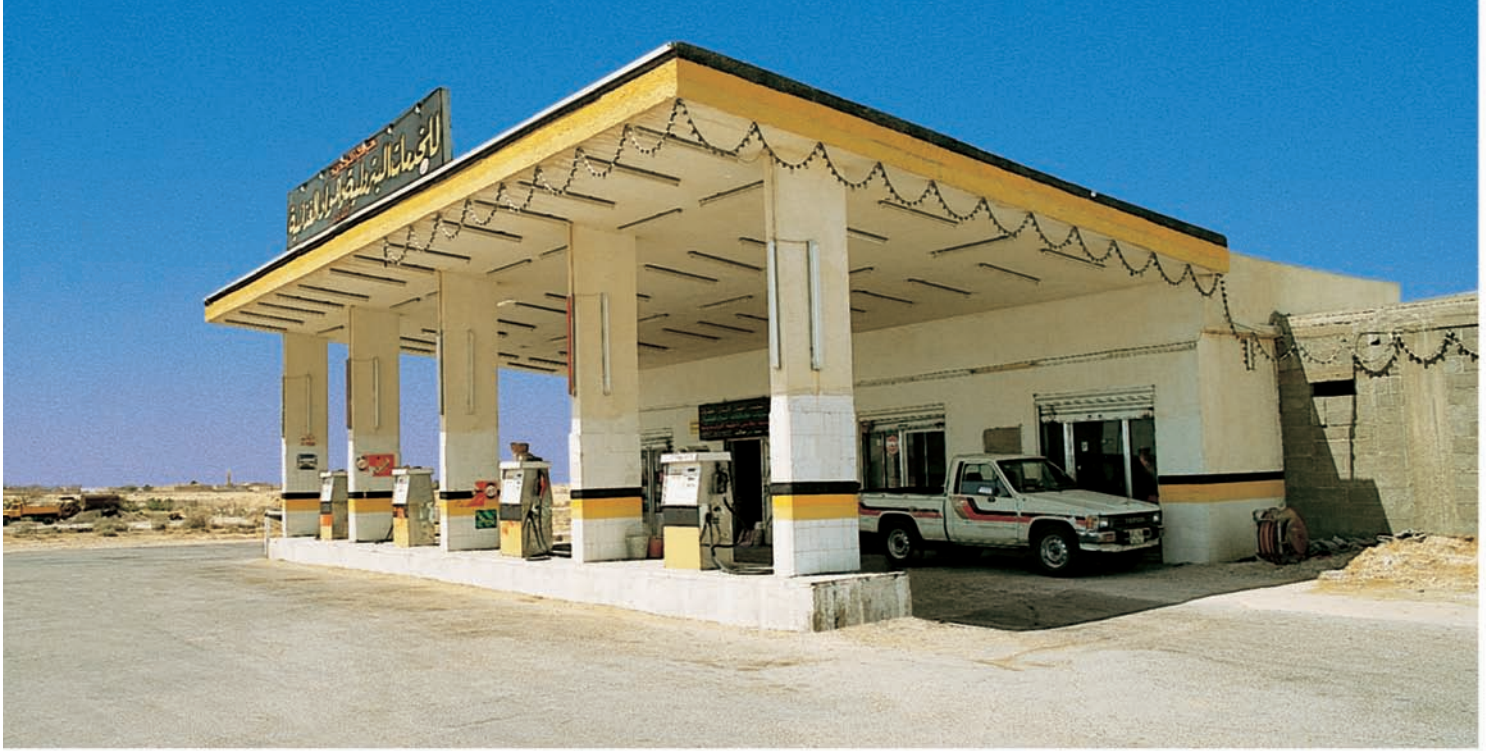
A petrol and services station in Raghbah
