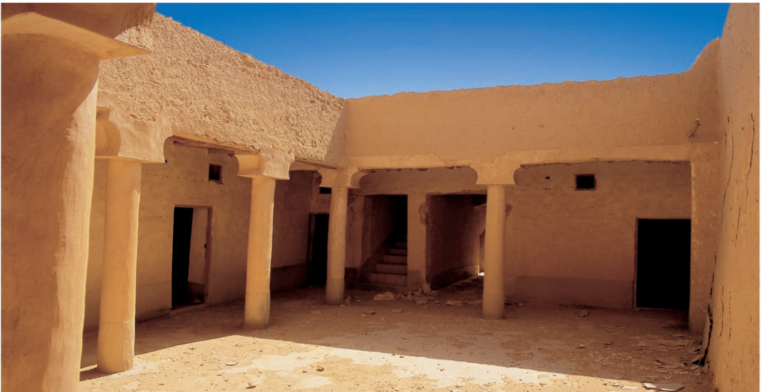
Misbeah ( roofed open gallery ) 'House B'
