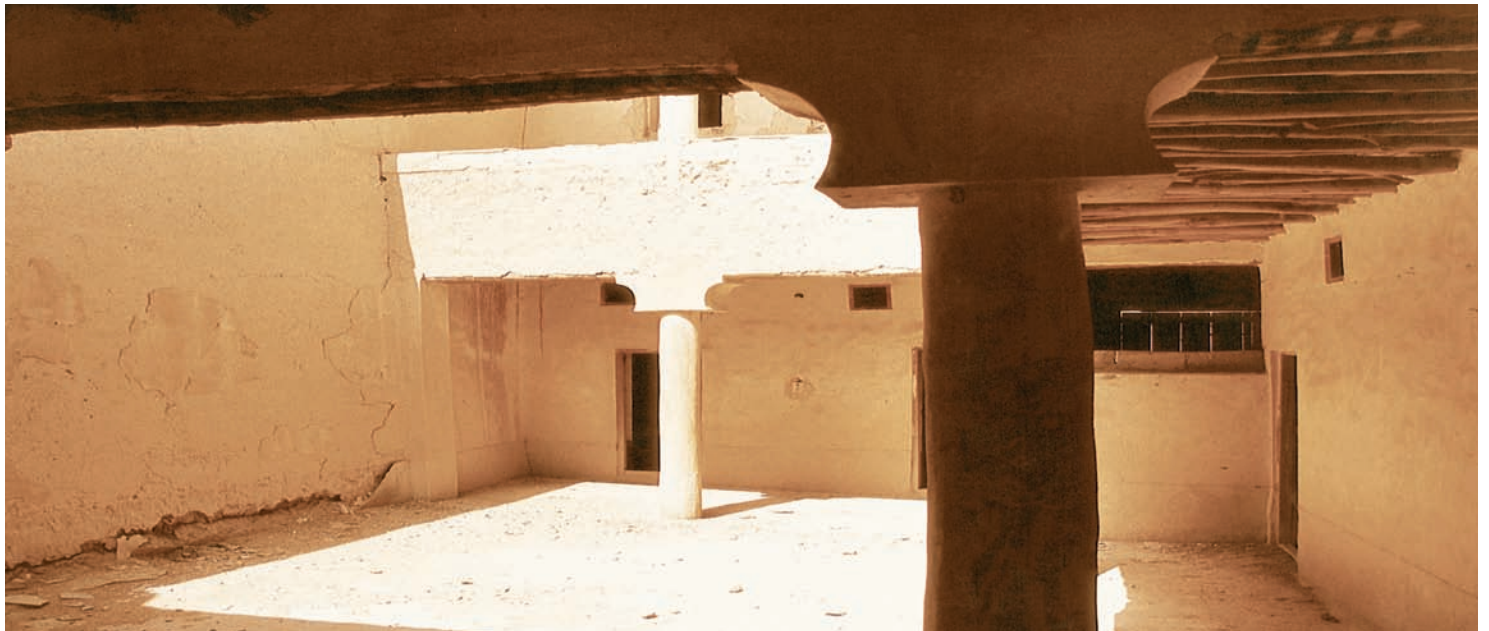
Loggia ( house A )
