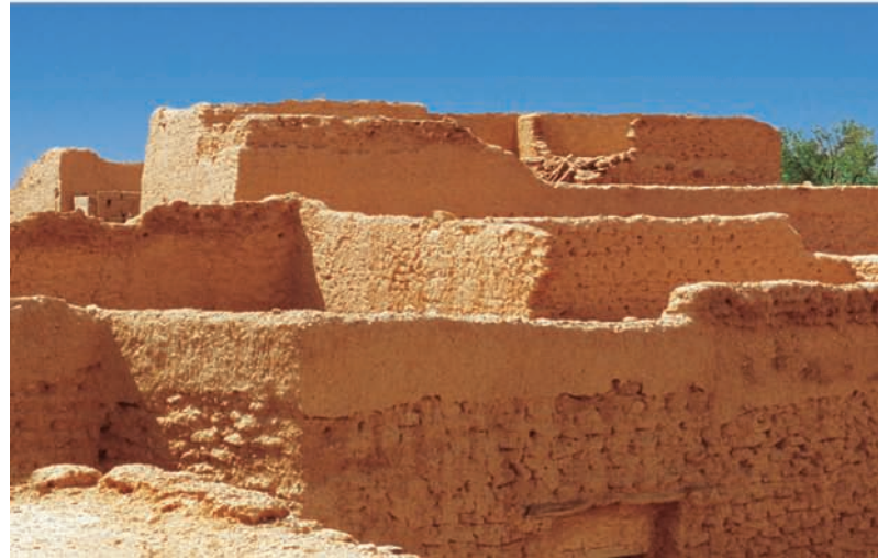
Same building in Nab'a Quarter
