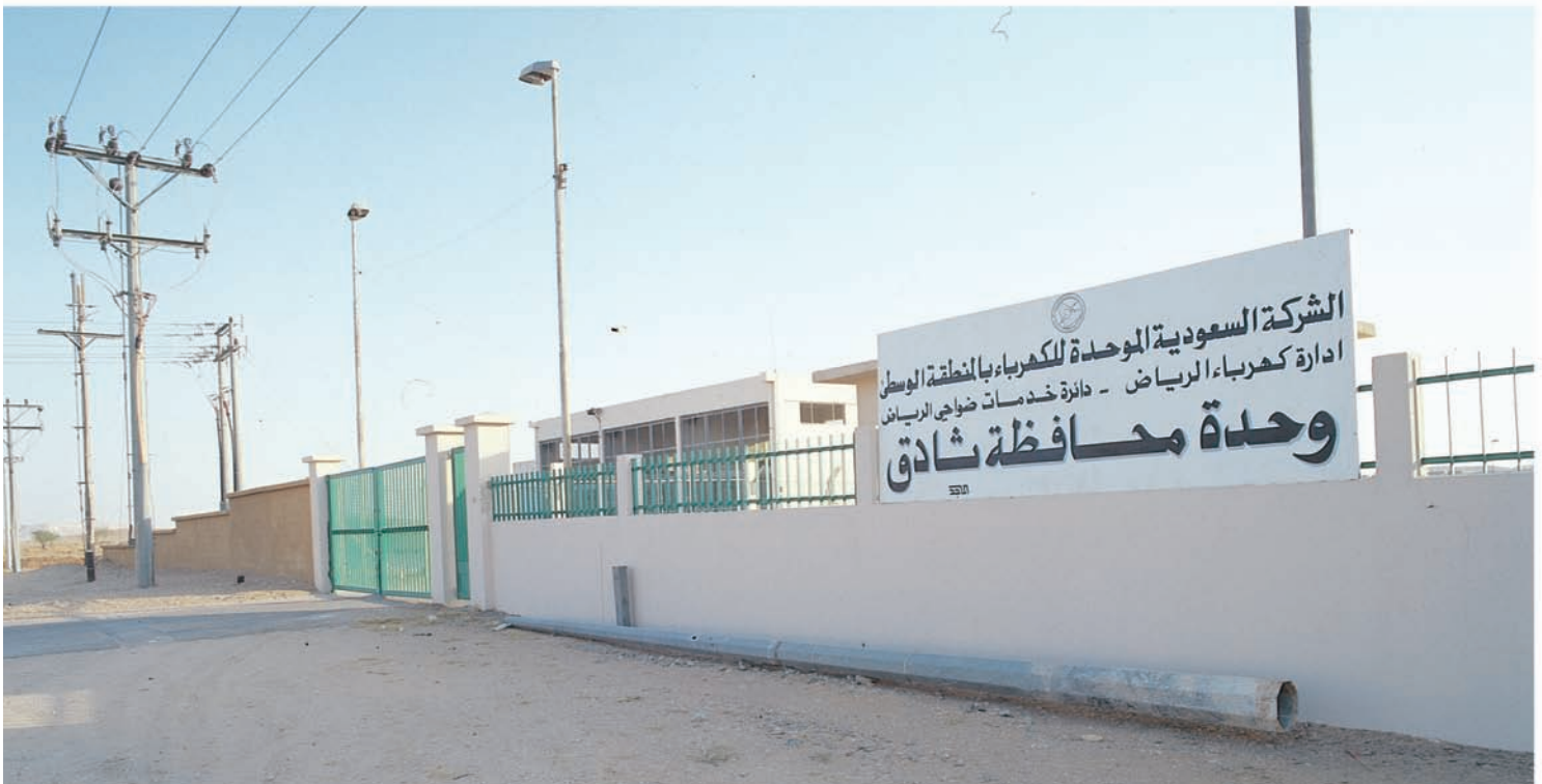
Thadeq Power Plant
